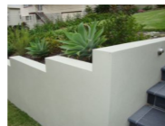
RW-01 Concrete Blockwork Retaining Wall with rendered finish
